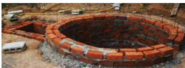
Figure 3: Installation of a biogas plant.
